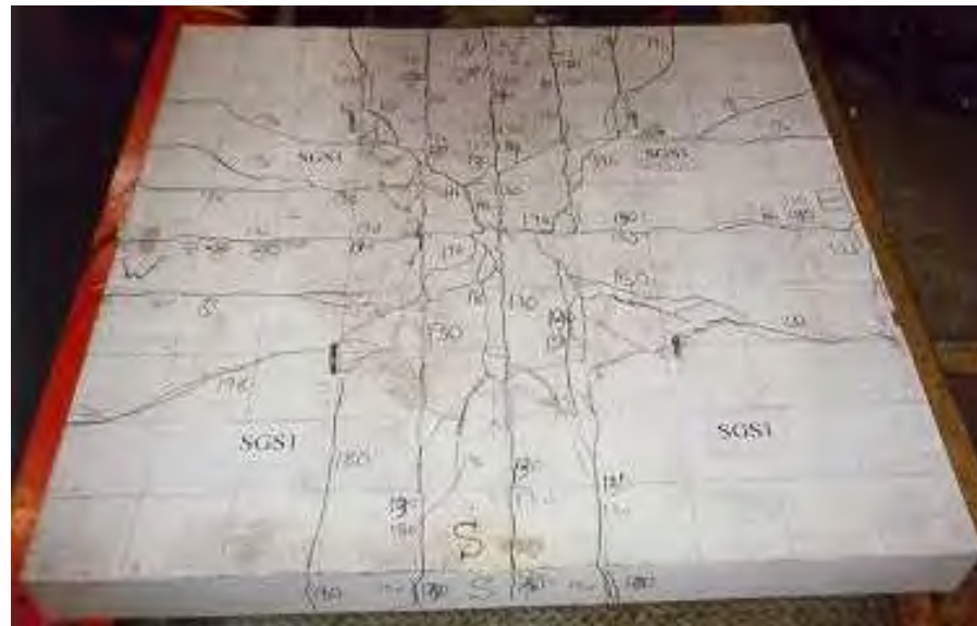
Slab SGS1 at Failure
