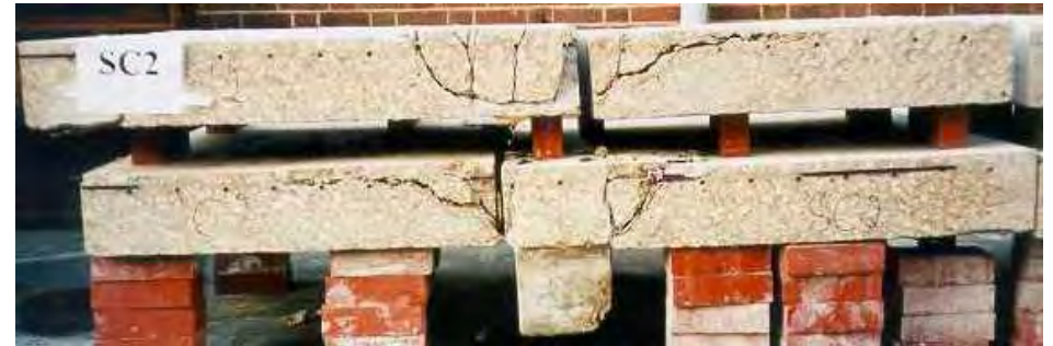
Section through Slab SC2 at Failure
