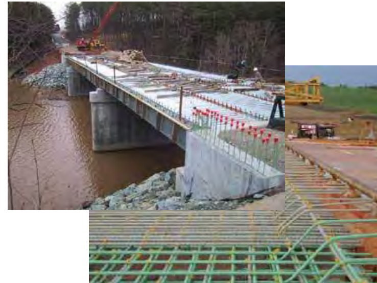
Use of GFRP for bridge deck construction (Franklin county bridge Virginia)
