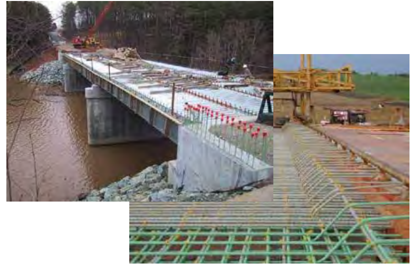
Use of GFRP for bridge deck construction (Franklin county bridge Virginia)
