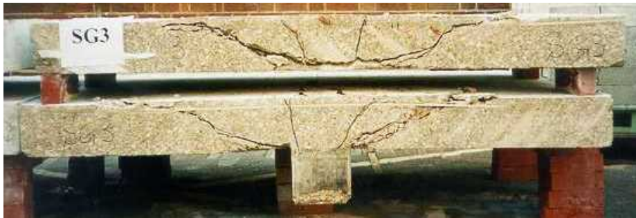
Section through Slab SG3 at Failure
