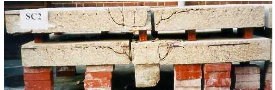
Section through Slab SC2 at Failure
