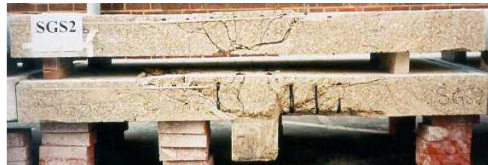
Section through Slab SGS2 at Failure
